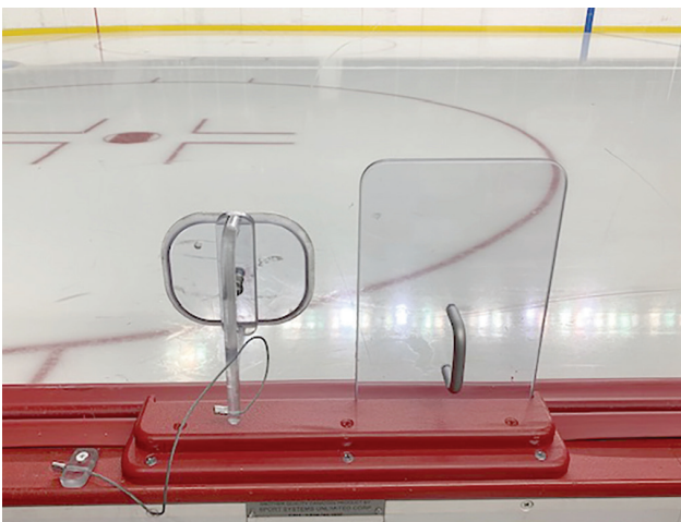
Removable and slide camera hole covers.
